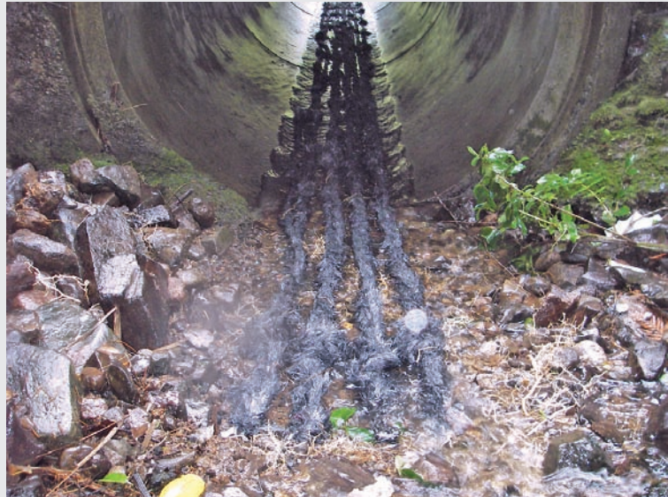
Textured ropes installed in a stream culvert to aid fish passage. Photo: Bruno David
